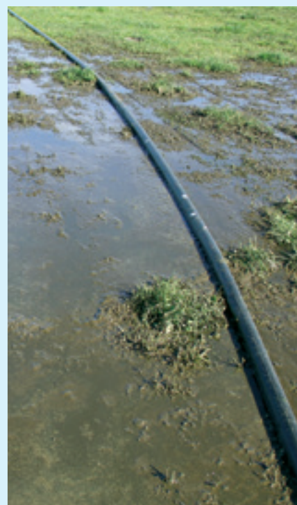
Ponding caused by effluent irrigation to land. This is a breach of the prohibited rules.
