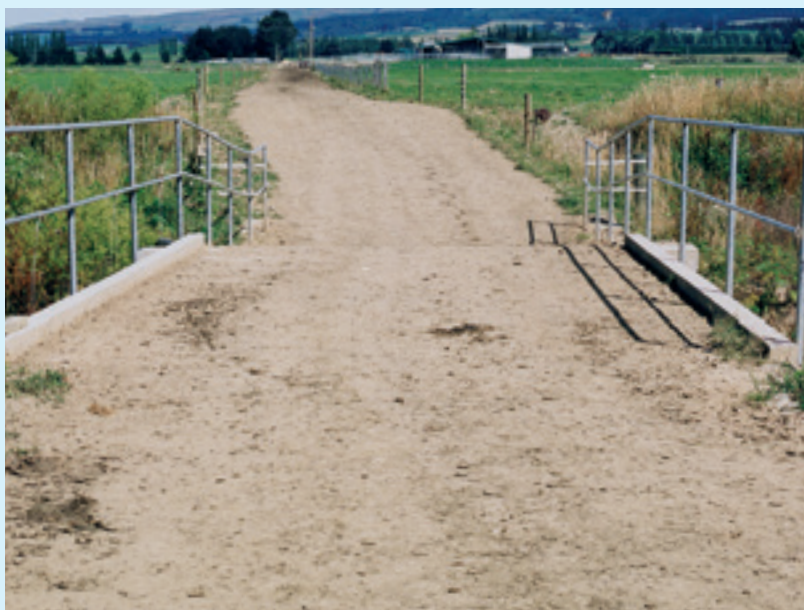
The installers of the bridges pictured have made use of the new water quality rules. The bridge on the right, which is used by stock, has a bund to stop animal waste entering the creek. The bridge on the left is not used by stock so does not require a bund.
