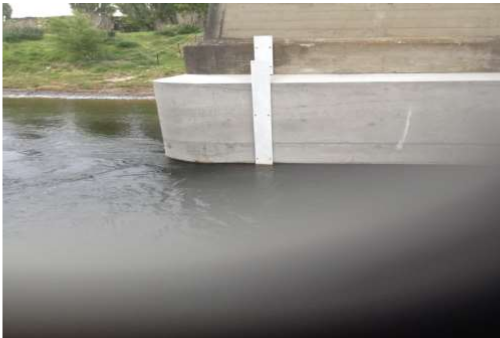
Figure 21 – Timber boards attached to a stable structure
