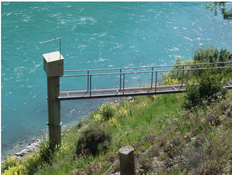
Figure 9– Catwalk (MWD design)
