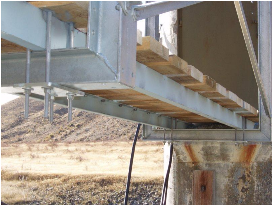
Figure 11 – Underside view of NIWA-design catwalk
