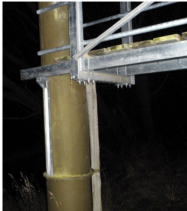
Figure 12 – Attachment to 600-mm stilling well with the new seat design (NIWA)
