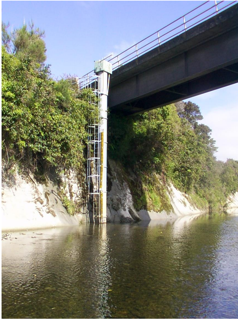
Figure 13 – Water level station showing multiple sections and housing Photographer: Evan Baddock.
