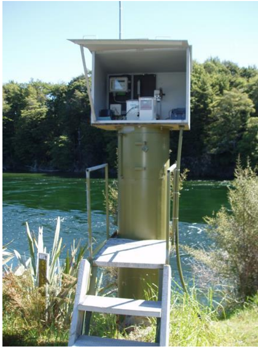
Figure 12 – Typical stilling well housing design Photographer: Evan Baddock.
